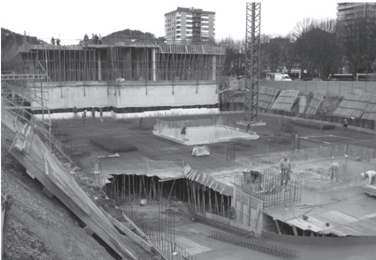
NanoGUNE's early construction works (December 2007).
